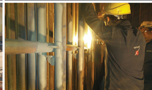
Boiler Tube Coating with CrCarbide-NiCr Cord
